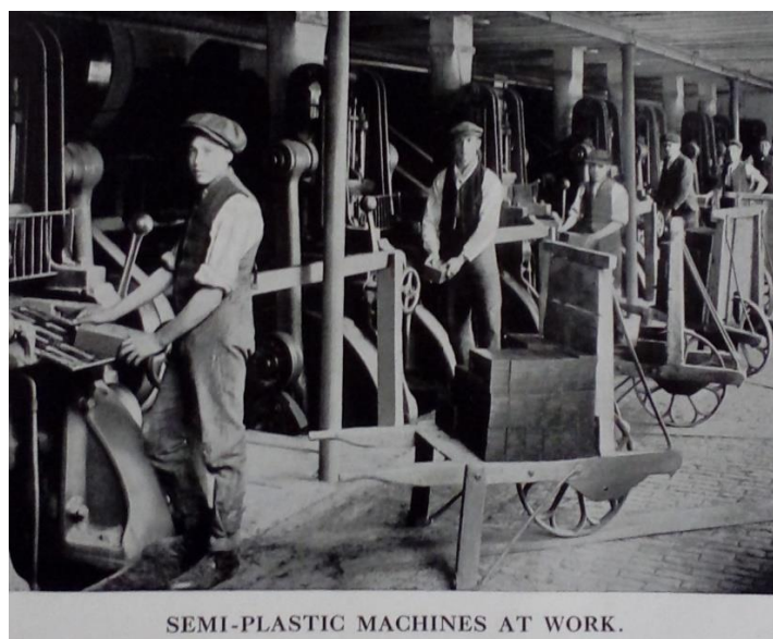
DDX 1866: Whittaker's brick making machinery at work
